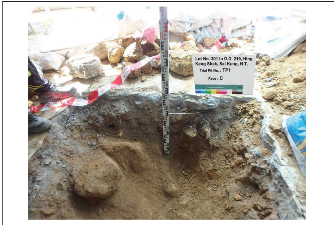
TRIAL PIT NO. TP1 FACE C
