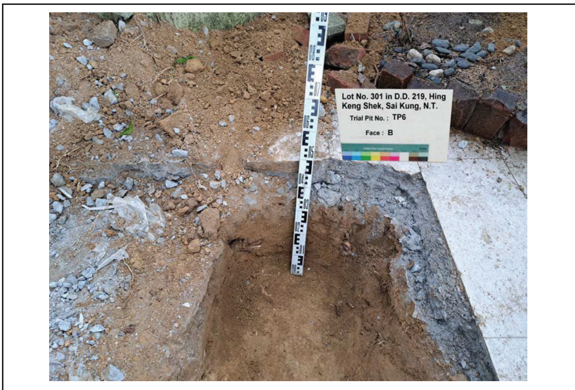
TRIAL PIT NO. TP6 FACE B
