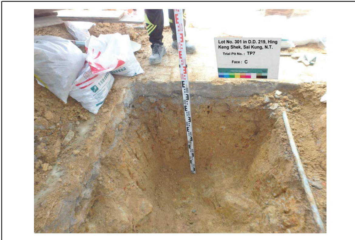
TRIAL PIT NO. TP7 FACE C
