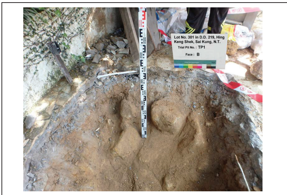
TRIAL PIT NO. TP1 FACE B
