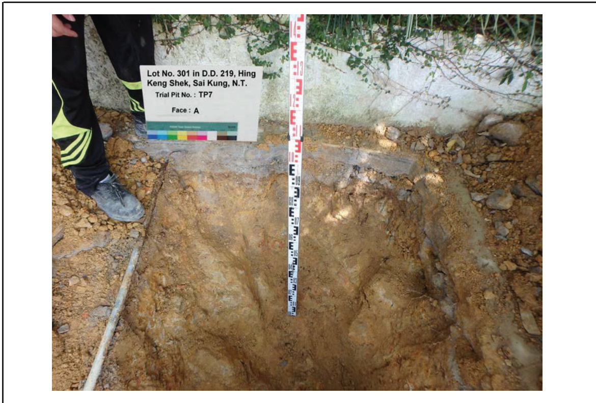
TRIAL PIT NO. TP7 FACE A
