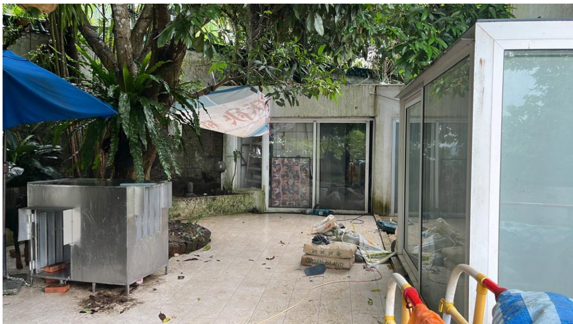
Photo V2 – General View of Central Portion of the Existing Building
