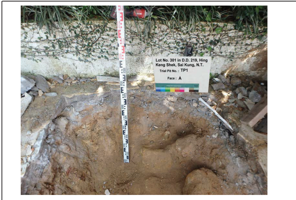
TRIAL PIT NO. TP1 FACE A
