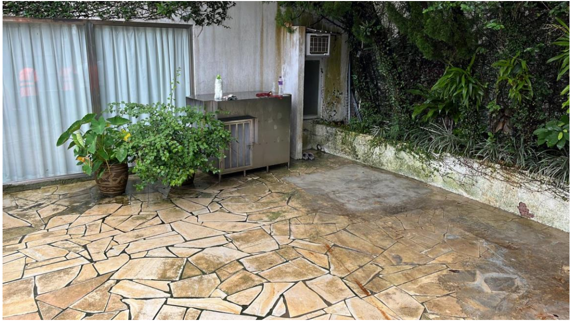
Photo V3 – General View of Northern Portion of the Existing Building
