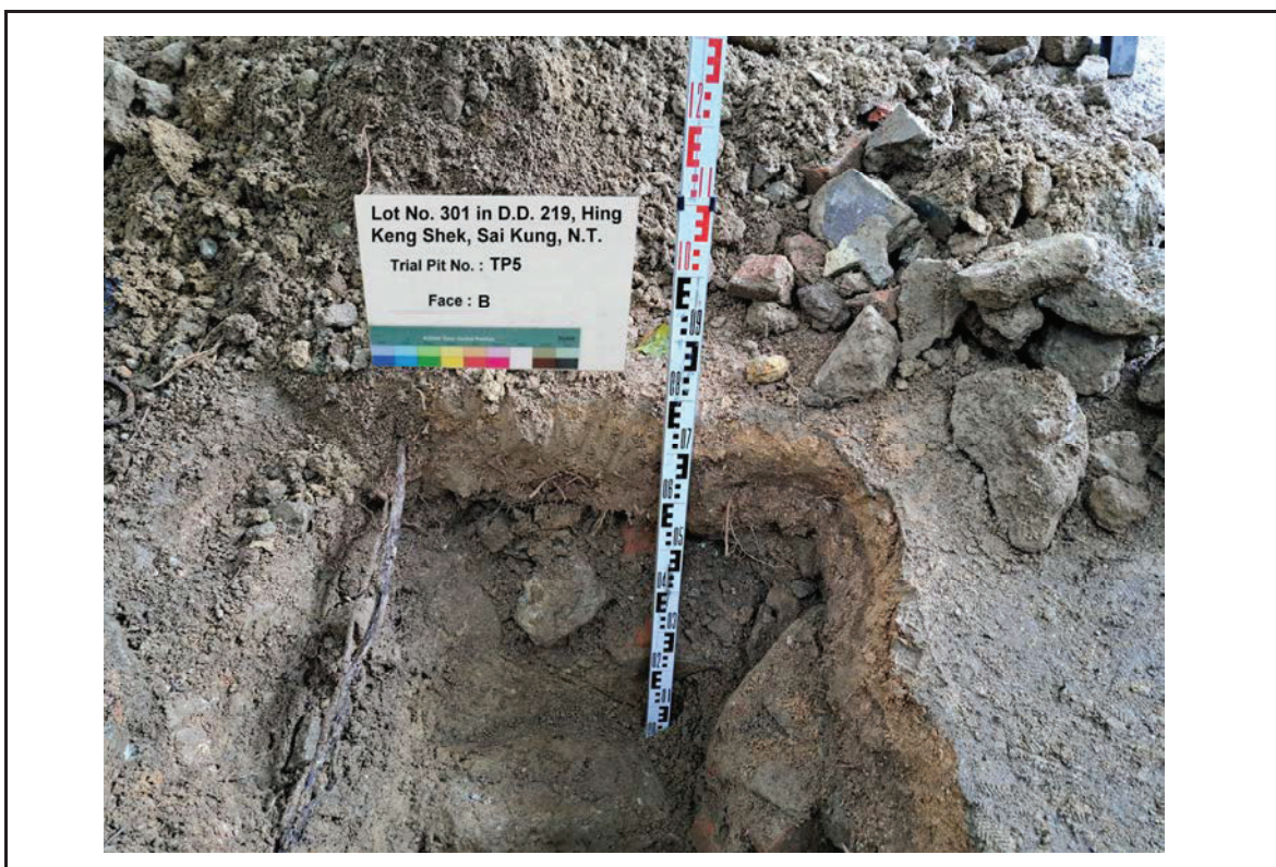
TRIAL PIT NO. TP5 FACE B
