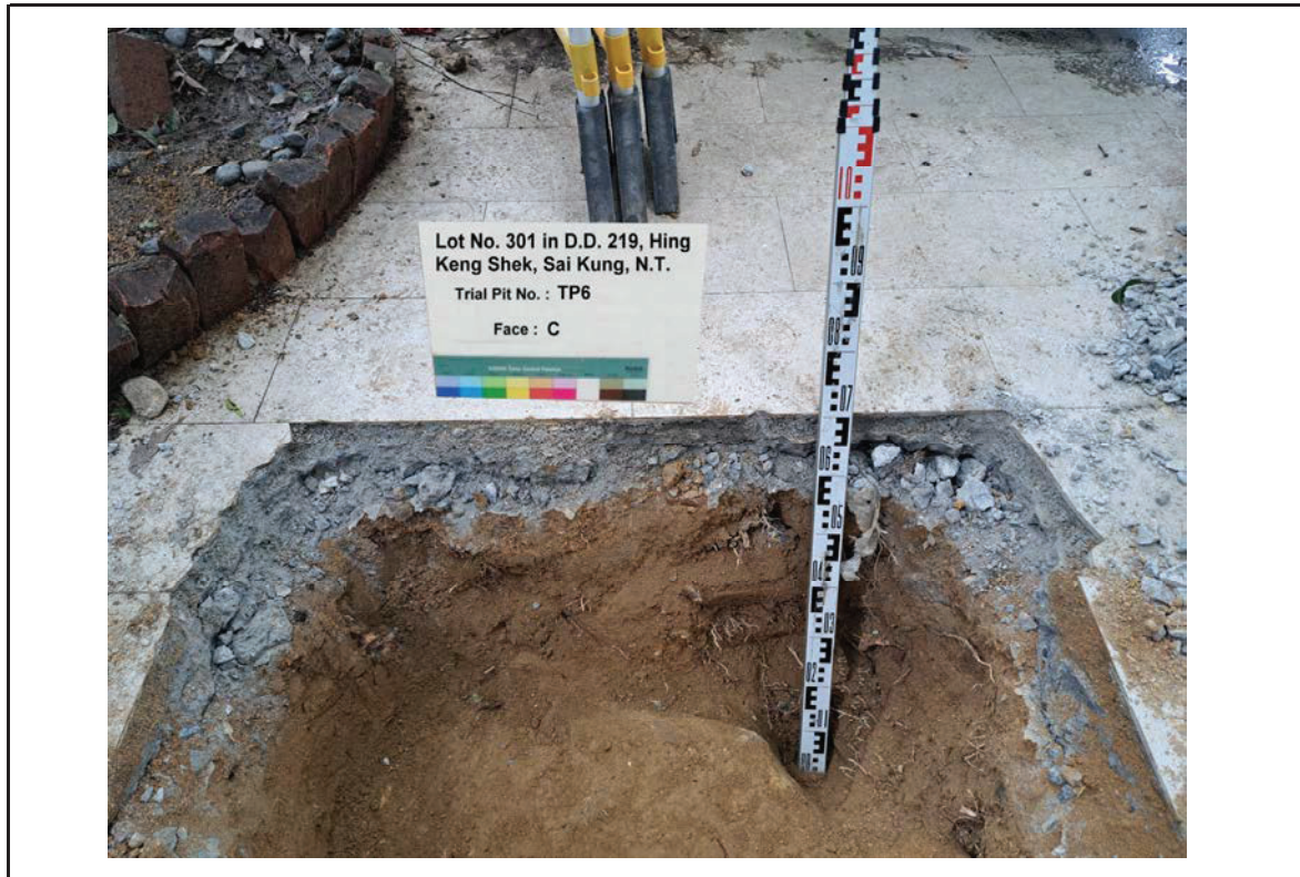
TRIAL PIT NO. TP6 FACE C
