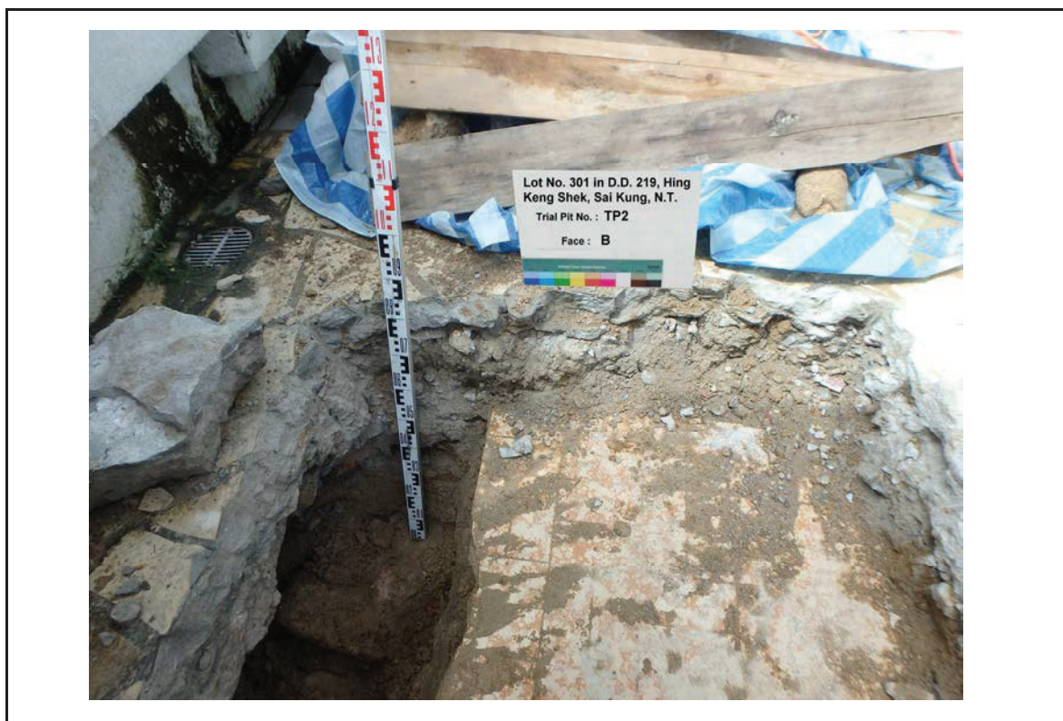
TRIAL PIT NO. TP2 FACE B
