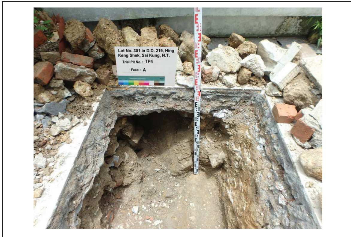
TRIAL PIT NO. TP4 FACE A
