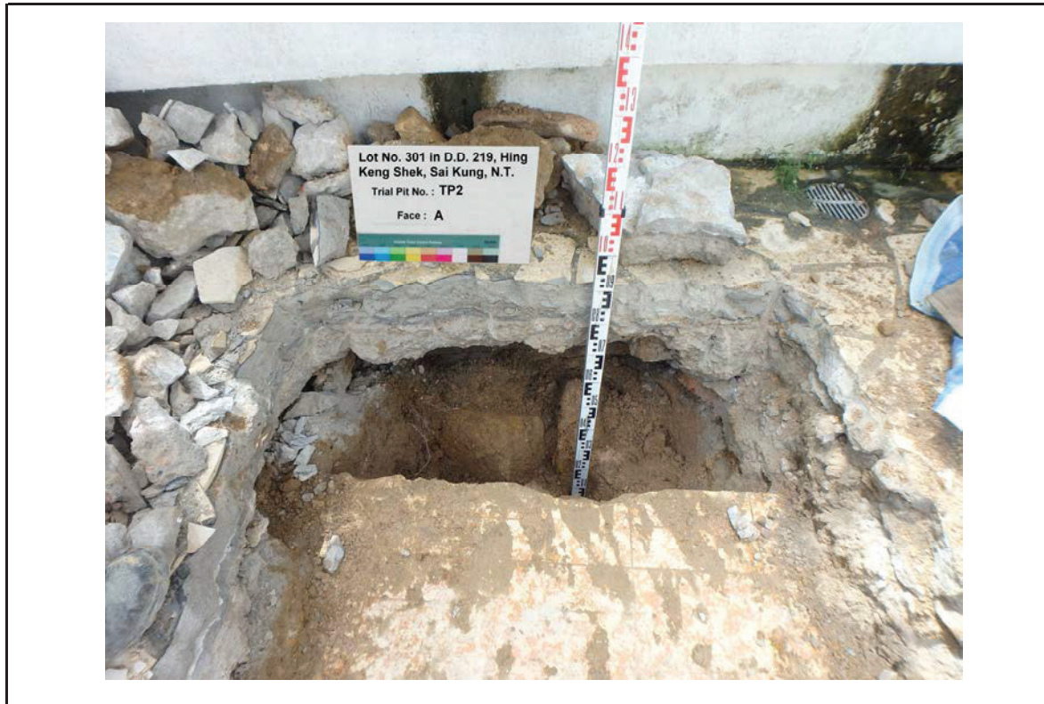
TRIAL PIT NO. TP2 FACE A
