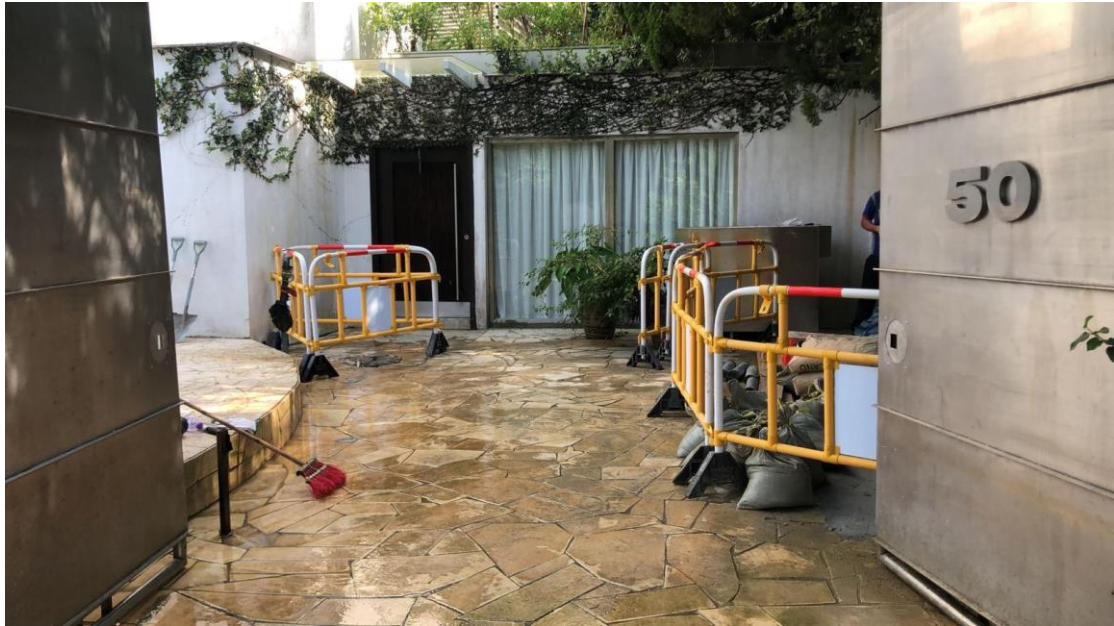
Photo V1 – General View of the Entrance to the Existing Building
