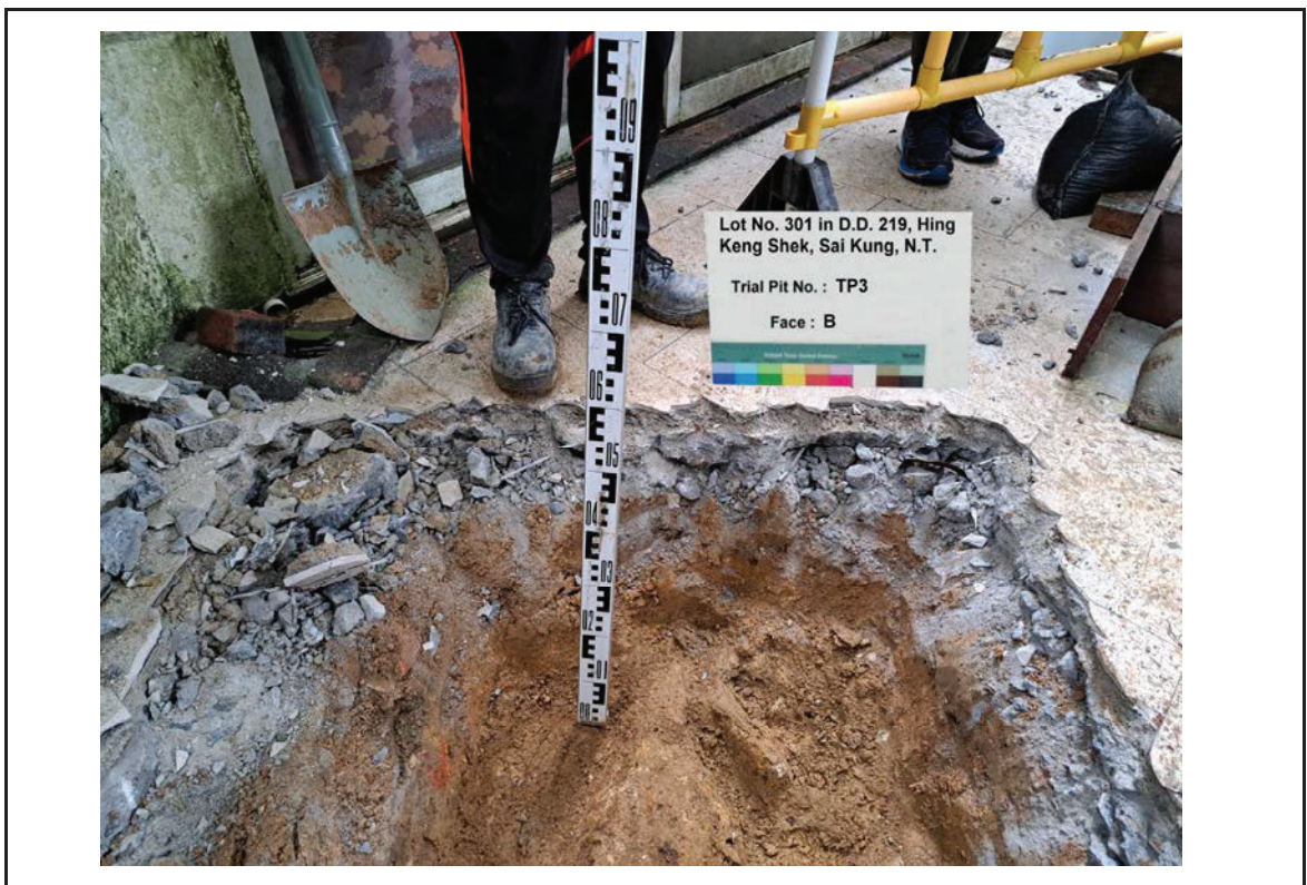
TRIAL PIT NO. TP3 FACE B
